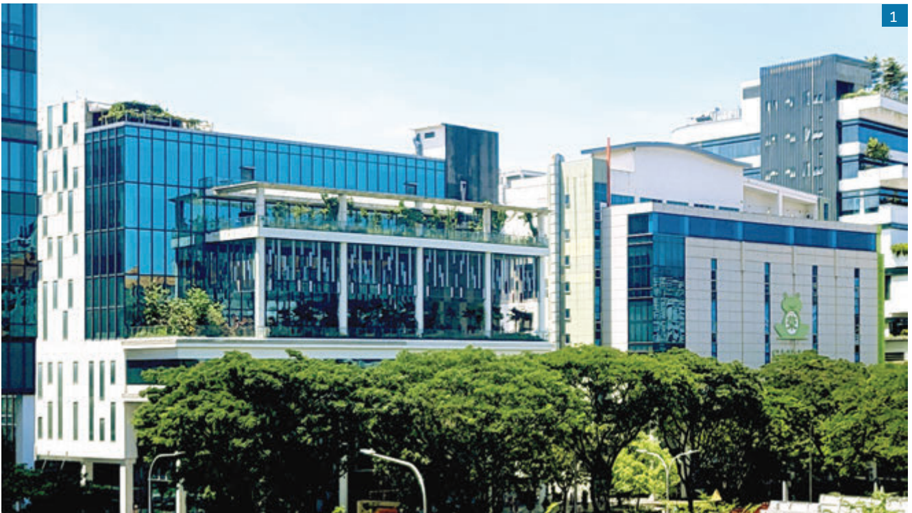
1. J'Forte Building, Singapore.
